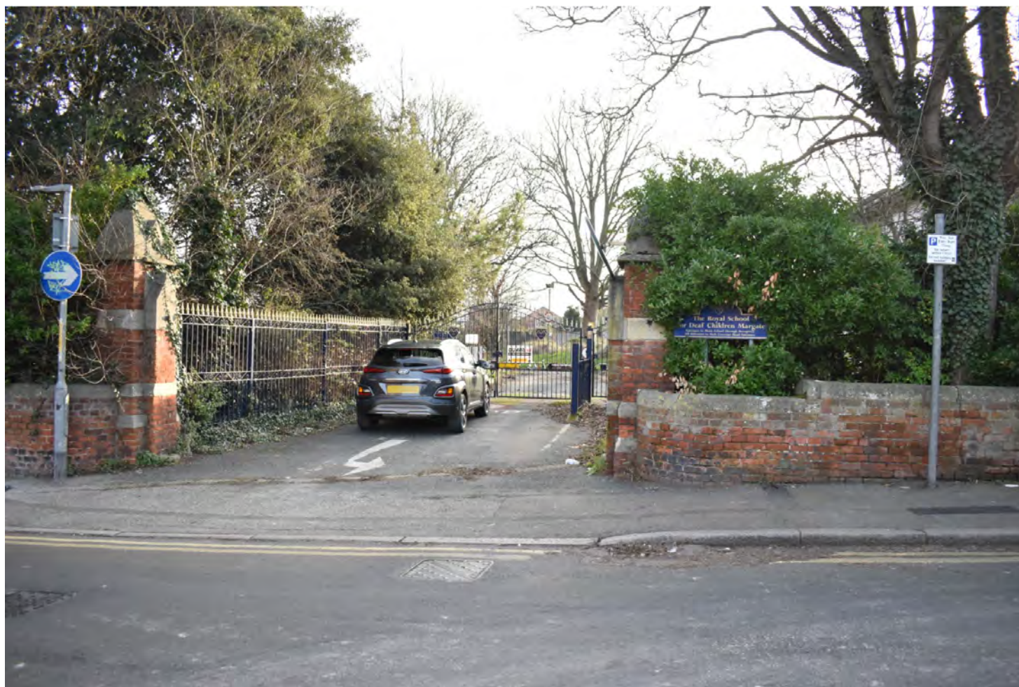
Plate 14: View of the main entrance (facing SE).
