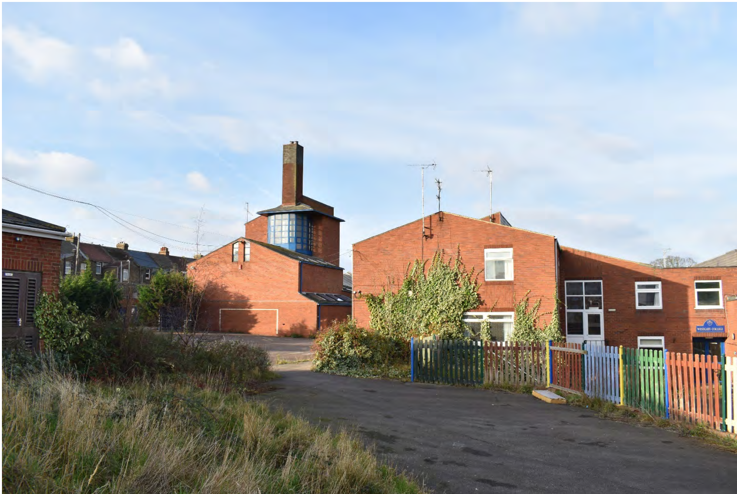
Plate 21: View at the south eastern end of the school buildings (facing SW)
