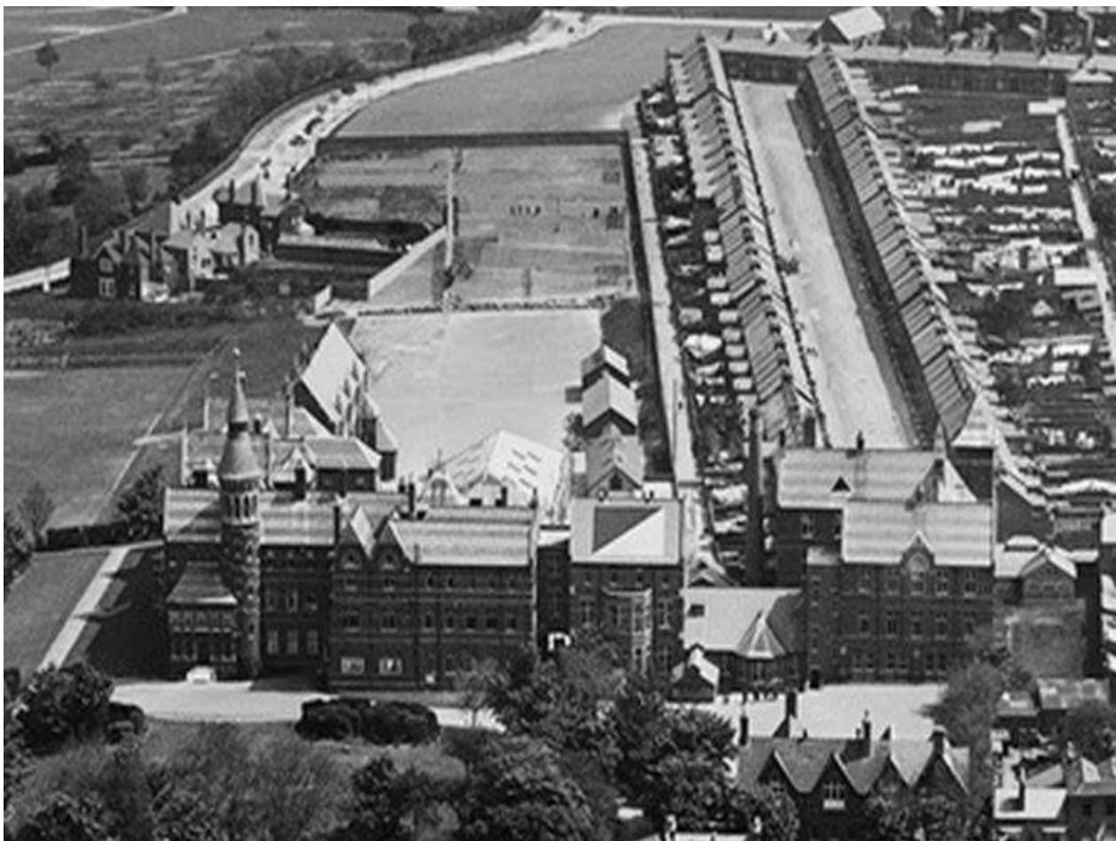
Plate 11: The School in 1920 (facing south east).
