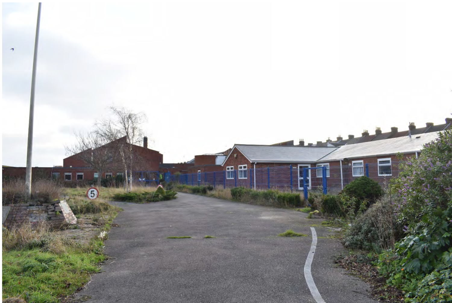
Plate 15: View to western end of the school buildings (facing SE).
